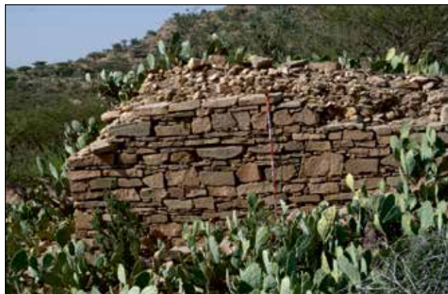
Figure 10: Abasa. Detail of constructive technique at a house
